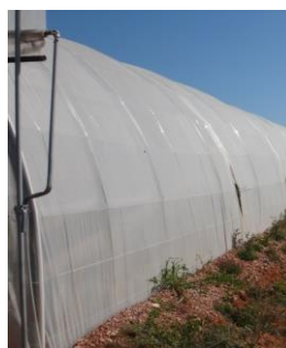
Tunnel blanchi – Photo CA 30
